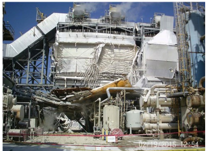
U.S. Chemical Safety Board Finds Multiple Safety Deficiencies Led to February 2015 Explosion and Serious Bear Miss at the Exxon Mobil Refinery in Torrance, California 1/13/2016 http://www.csb.gov/exxonmobil-refinery-explosion/ , 30.03.2016
